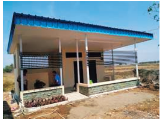
Completed toilet facilities
